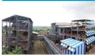
Resin Facility - Water and non-water
