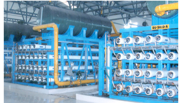
DEMINERALIZATION PLANTS FOR THERMAL POWER STATION
