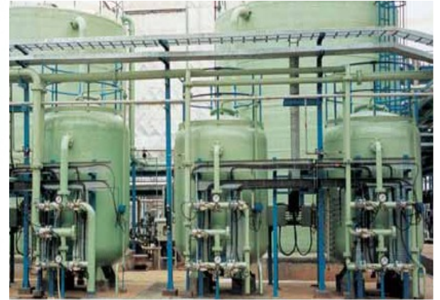
DEMINERALIZATION PLANTS FOR THERMAL POWER STATION
