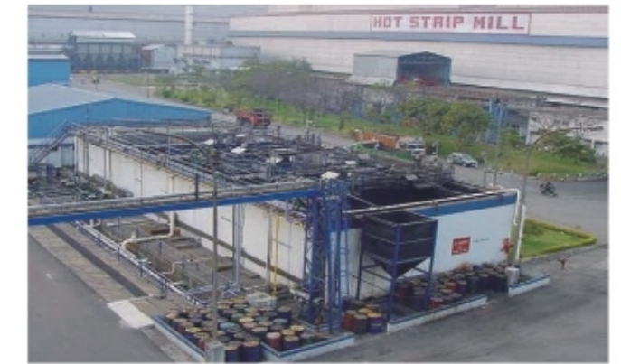
Complete water and waste water treatment at Tata Steel
