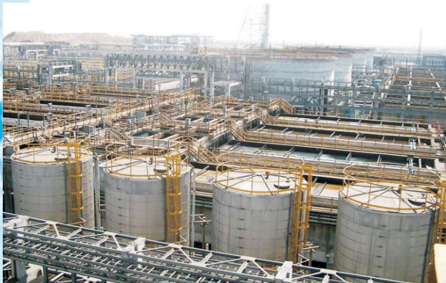
Slop oil tanks
