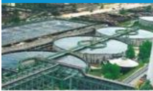
EOU & Engineering Design Facility
