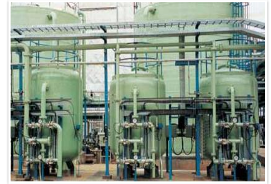
Demineralization Plant for thermal power station
