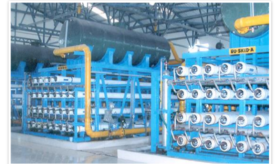
Demineralization Plant for thermal power station
