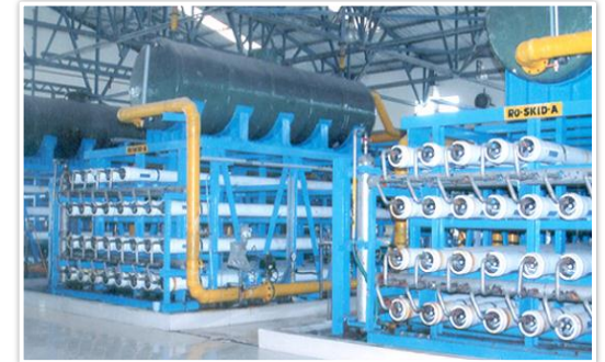
Demineralization Plant for thermal power station
