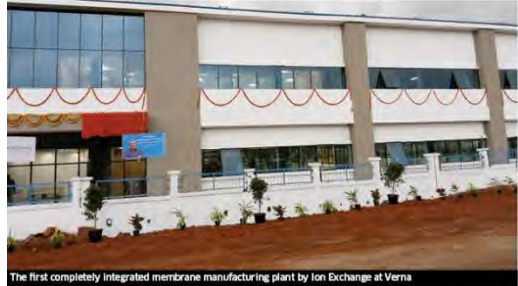
The first completely integrated membrane manufacturing plant by Ion Exchange at Verna
