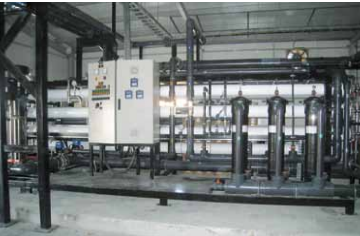
2 x 300,000 USGPD (2 x 1135 m 3 /d) brackish water treatment reverse osmosis plant supplied to Umm Al Quwain, Government of UAE
