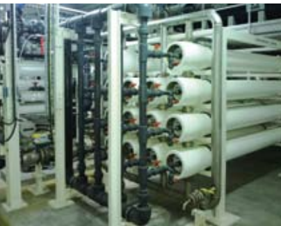
Ion Exchange is undertaking the O&M of this 3840 m 3 /day RO plant at Faud site, Sultanate of Oman
