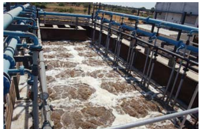
Membrane bio-reactor section
