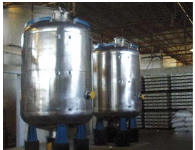
Two SS 316 activated carbon filters for Pepsi Bottling Plant, Bahrain.
