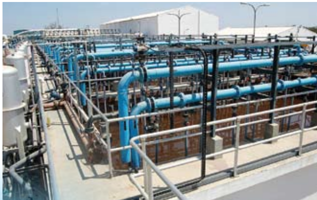
Membrane bio-reactor
