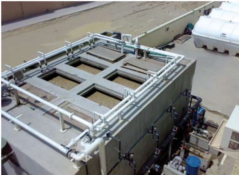
Membrane bio-reactor
