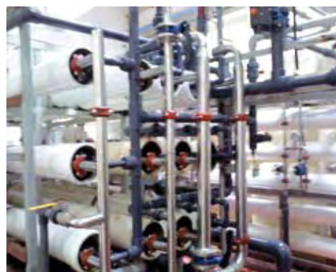
Refurbishment of packaged drinking water treatment plant for Coca Cola, UAE
