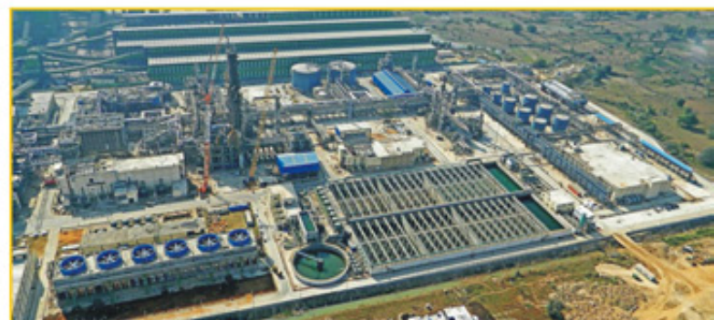
Effluent treatment plant at a steel complex
