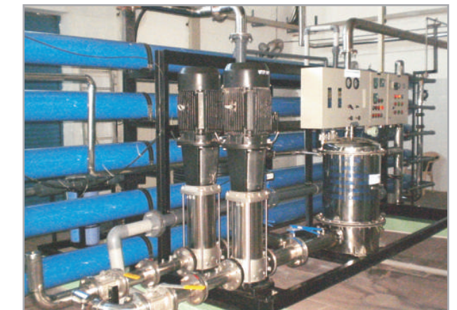
Treatment system at Pearl Drinks, Noida, comprising multigrade and activated carbon filtration (dechlorination), reverse osmosis and activated carbon filtration (for pesticide removal), micron filtration and ultra violet. The water produced is used to make carbonated beverages of Pepsi and complies with all the requisite beverage standards.
