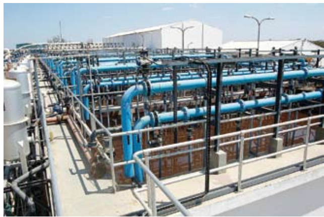
Membrane bio-reactor
