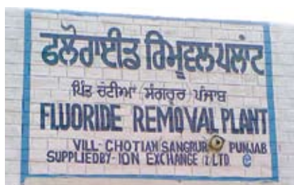
Our 2000 l/h fluoride removal system was installed at Chotian (Sangrur) village, Punjab
