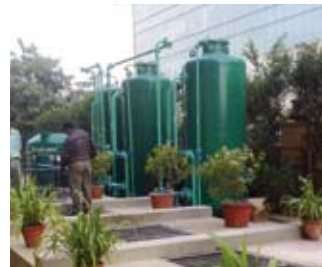
For Landmark Construction, Chennai, 10 m 3 /day NGPSTP
