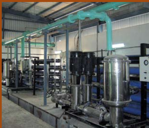
2 x 80 m 3 /h ultrafiltration and reverse osmosis plants to treat river water at Tamil Nadu Newsprint and Papers Ltd., Karur, Tamil Nadu.
