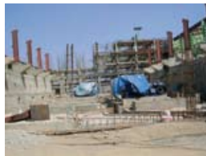
Furnace Skid CT
