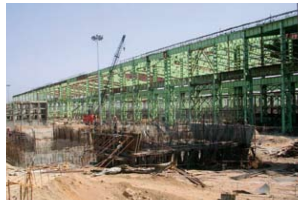
Overall View of Utility Water System during construction
