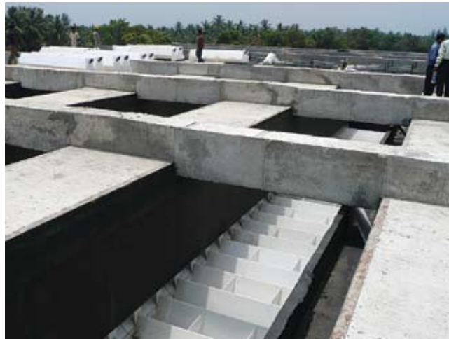
Upflow Anaerobic Sludge Blanket (UASB)
