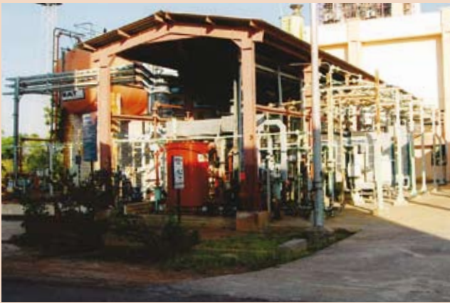
Auto demineralisation plant at ST-CMS, Neyveli, Tamil Nadu
