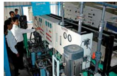
Inspection team conducts O&M audit of plant
