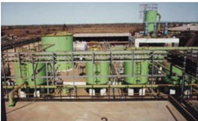
cooling water storage tank and multigrade sand filter.
