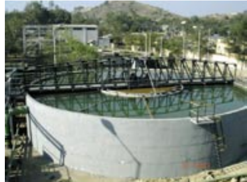
At INDAL Hirakud, 550 m 3 /h pretreatment plant consisting of high rate solids contact clarifier and a 20 m 3 /h DM plant with pressure sand and activated carbon filters, strong acid cation, strong base anion and mixed bed units.
