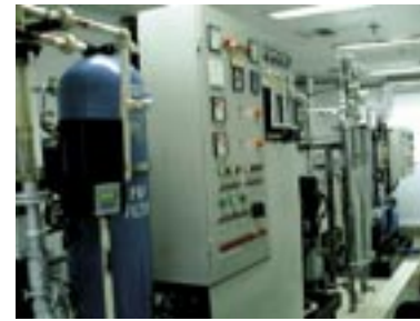
At Johnson & Johnson, Mumbai modification of competitor-supplied RO-polisher unit from 200 to 600 LPH, including addition of six SS pressure vessels and twelve HSRO membranes.
