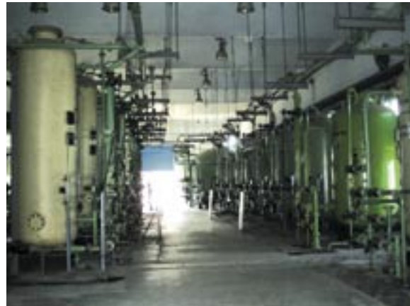
At INDAL Hirakud, 550 m 3 /h pretreatment plant consisting of high rate solids contact clarifier and a 20 m 3 /h DM plant with pressure sand and activated carbon filters, strong acid cation, strong base anion and mixed bed units.
