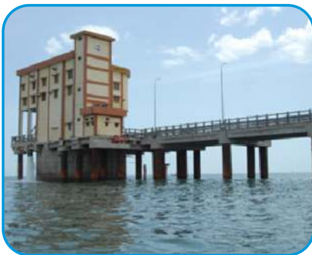
Sea Water Intake Plant
