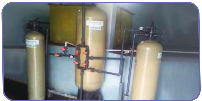
INDION ® Fluoride Removal Tube Well attachment, Madhya Pradesh
