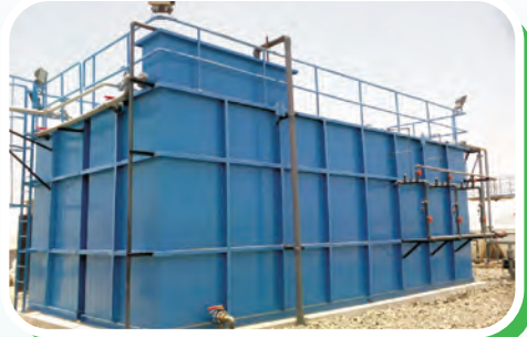
Membrane bioreactor at a construction company
