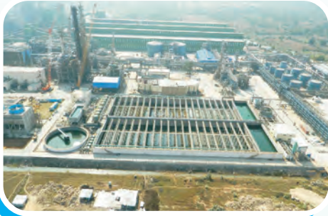
Effluent treatment plant at a steel industry
