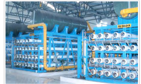
Demineralization Plant for thermal power station
