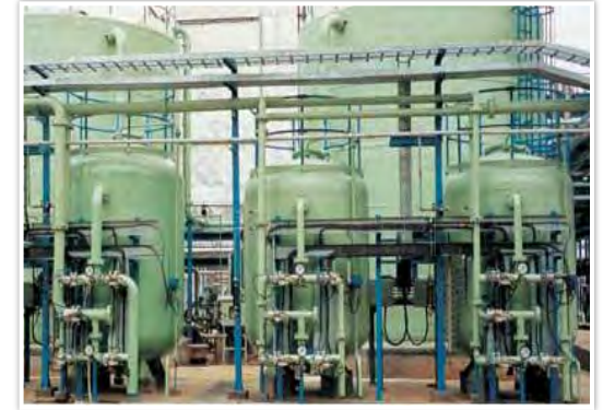
Demineralization Plant for thermal power station
