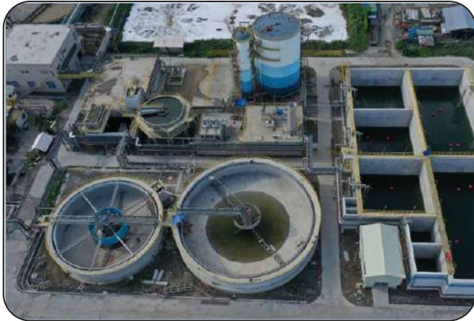
Birds eye view of complete Waste Water Treatment System for a leading paper manufacturer
